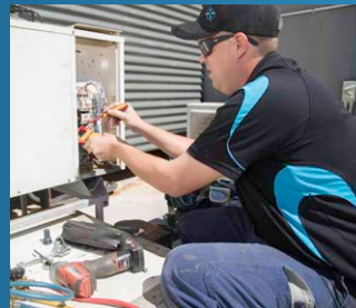
Repairs & Maintenance on Coolrooms
