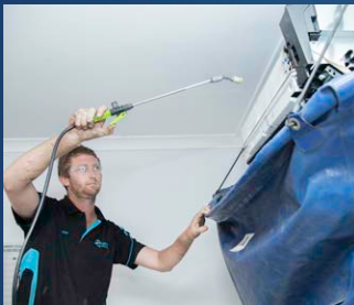
Servicing & Repairing Air Conditioners
